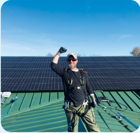
Nashua, NH Lake St. Fire Station
